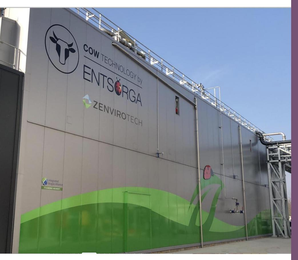
THE COW SEMI-DRY SYSTEM, BASED ON A DEDICATED PRETREATMENT AND A SEMY DRY PLUG FLOW DIGESTER, IS ONE OF THE MOST INNOVATIVE GREEN TECHNOLOGIES FOR THE RECOVERY OF BIOGAS FROM ORGANIC WASTE ON THE MARKET.
