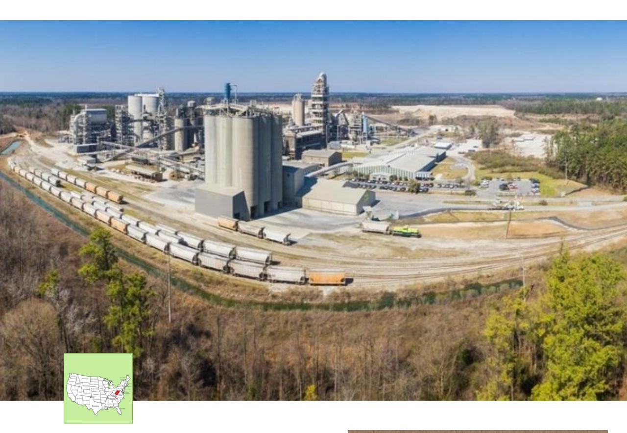
A DOUBLE IMPORTANT PROJECT THAT CREATED WITH ARGOS CEMENT, WHICH TESTIMONIES THE PROJECT FINANCING CAPACITY OF ENTSORGA. ARGOS CEMENT USE ENTSORGA PELICAN™ FEED LINE FOR THE CONTINUOUS FEEDING AT ITS CEMENT KILNS WITH ENTSORGA PROMETHEUS™, THE ALTERNATIVE FUEL PRODUCED IN THE ENTSORGA WEST VIRGINIA PLANT, NEAR THE CEMENT PLANT.
