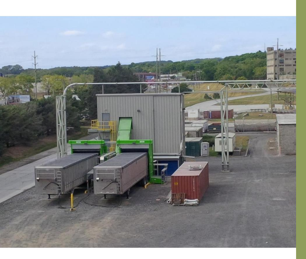
ENTSORGA'S PELICAN<sup>TM</sup> SYSTEM PROVIDES A COMPLETE LINE FOR THE SUPPLY OF ALTERNATIVE FUELS TO CEMENT KILNS
