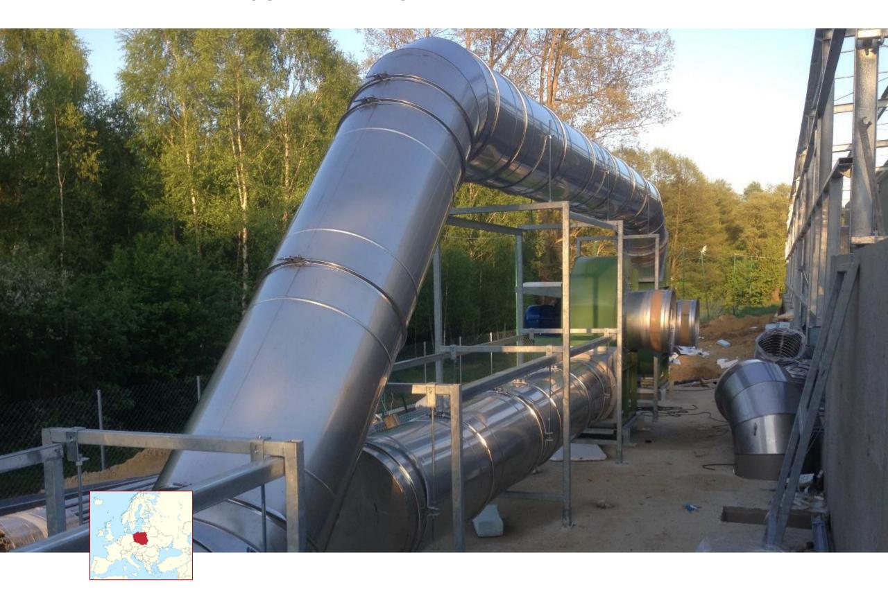
THE MBT PLANT IN SIEDLCE, POLAND, USES THE ENTSORGA FORCED AERATION SYSTEM. HEART OF THE PROCESS OF BIOSTABILIZATION, THE SYSTEM ALLOWS TO ACCELERATE THE REACTION IN A CONTROLLED AND EFFICIENT WAY, TO OBTAIN A STABLE REJECTION, WITH VERY LOW MOISTURE CONTENT, SUITABLE FOR THE LANDFILL IN ACCORDANCE WITH THE TERMS OF LAW.
